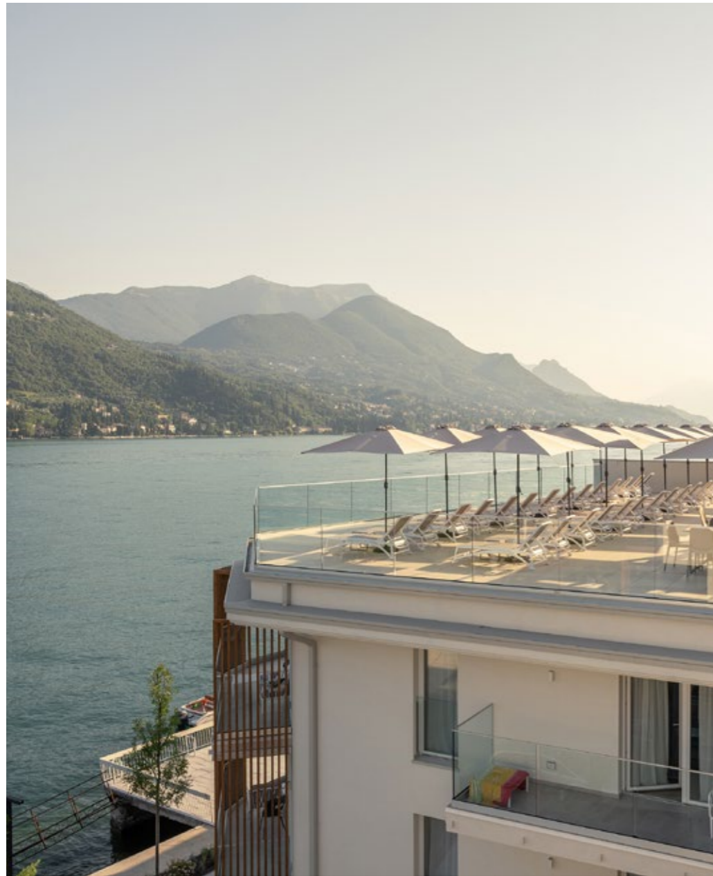
AH Porticcioli Boutique Apartments Resort San Felice del Benaco - Italy Project: Hotel Products: Atlantico, Pop
